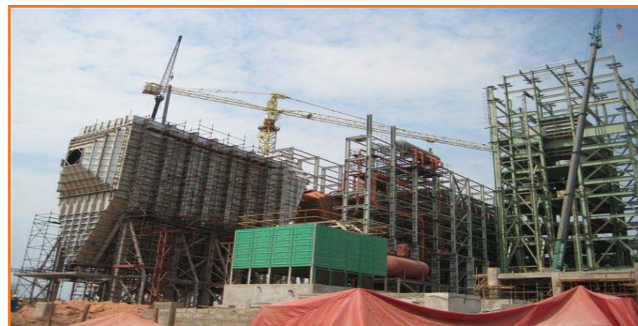
View of ESP, Boiler, Smelter building
