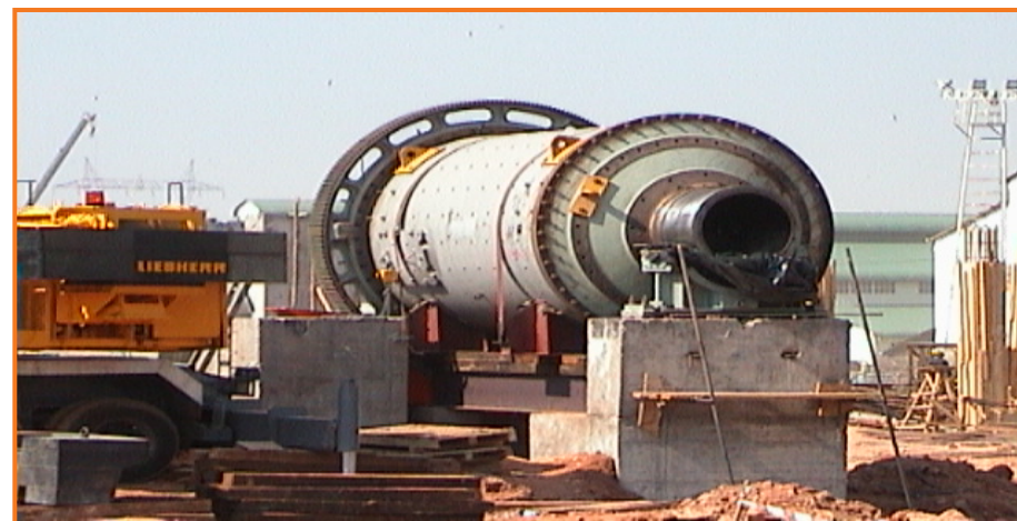
Concentrator-Regrind mill under construction
