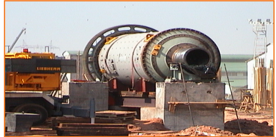
Concentrator-Regrind mill under construction
